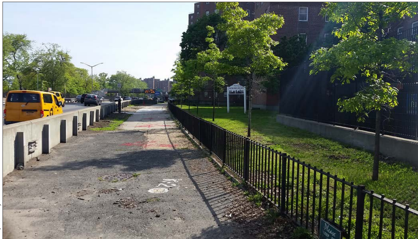
View of acquisition area along FDR Drive from north 3
