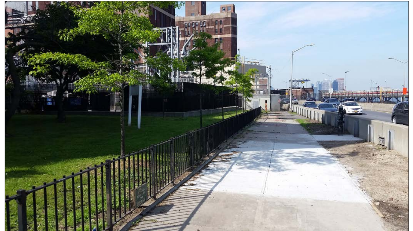
View along FDR Drive near center of acquisition area 2
