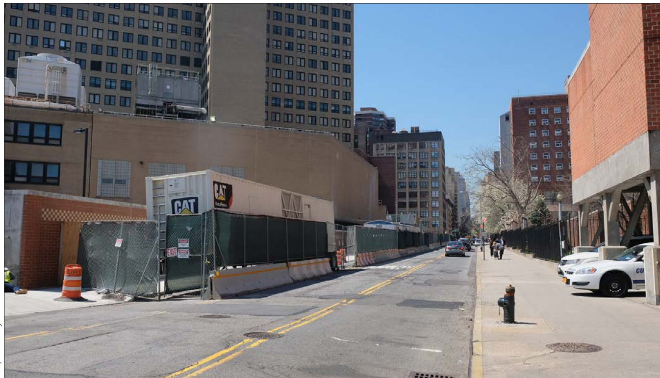
Northwest view of VA Hospital wall along East 25th Street 3
