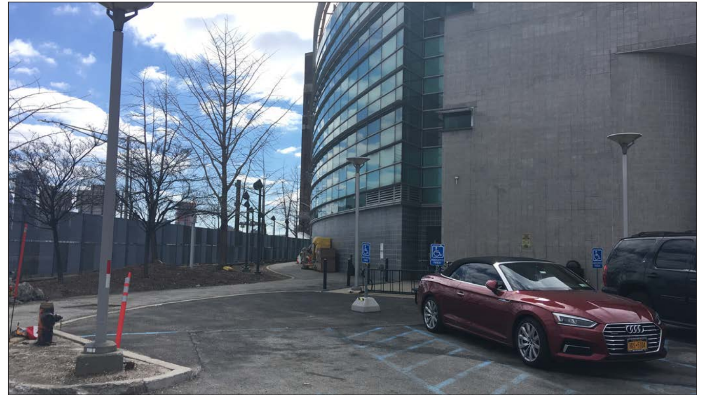
View south at Con Edison office building 2
